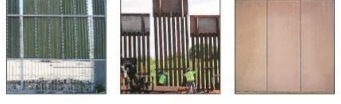
(From left) An existing barrier in El Paso sector of the US-Mexico border; a replacement barrier made of steel slats is installed in Naco, Arizona; a concrete wall is one of the prototypes commissioned by President Trump.
