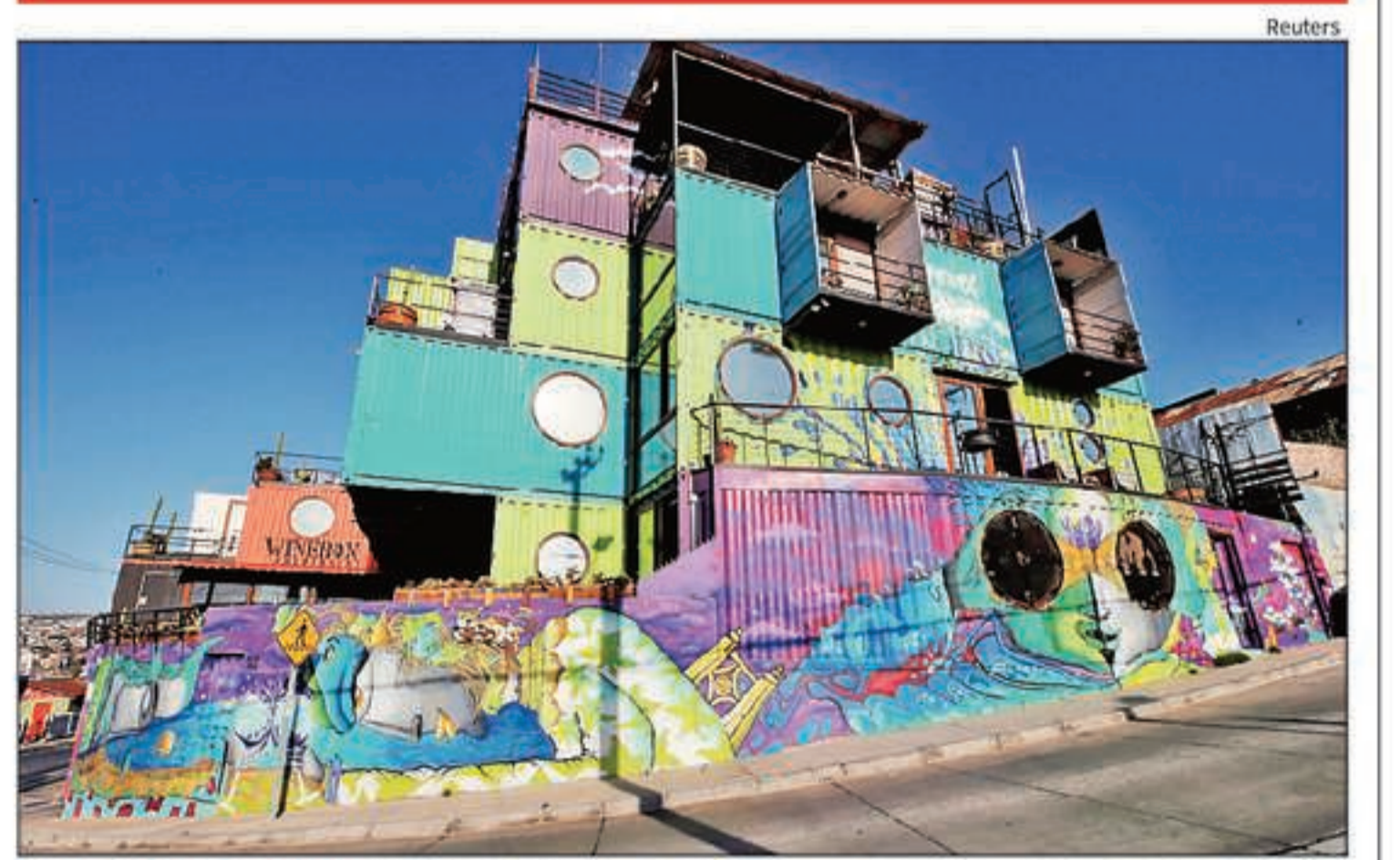
THINK INSIDE THE BOX: A hotel built with discarded shipping containers in Valparaiso, Chile
