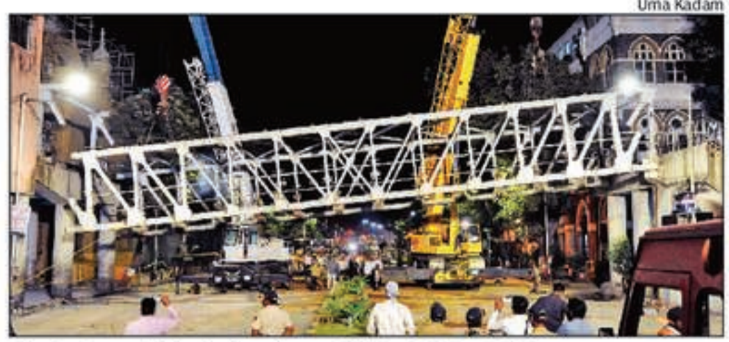
The foot overbridge being dismantled by BMC on Friday
