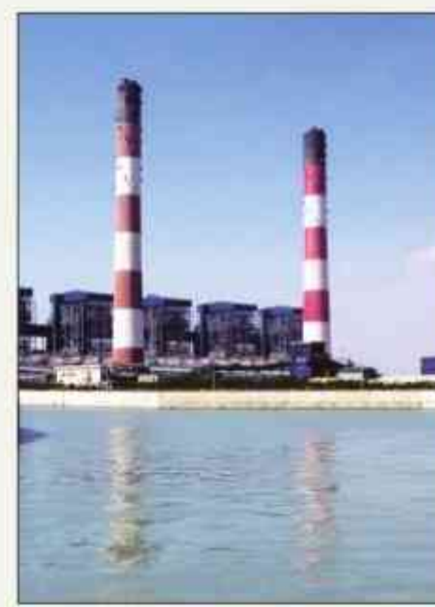
The power plant in Kutch. Express
