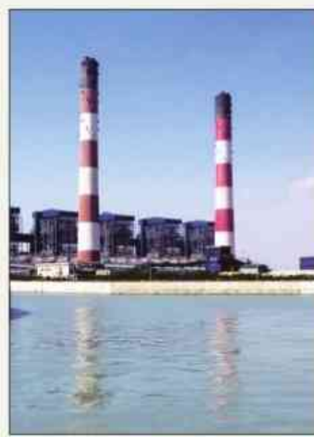
The power plant in Kutch. Express
