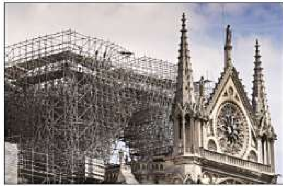
Damage seen on the facade at the Notre Dame Cathedral. AP
