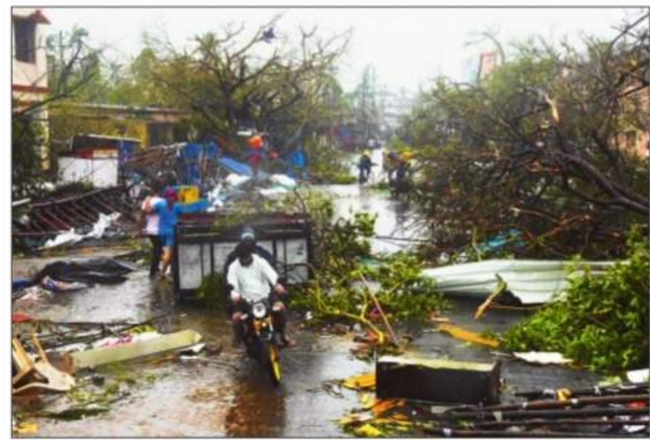
Even as human deaths have been averted to a very large extent, there is no running away from the destruction caused by Cyclone Fani. Reuters
