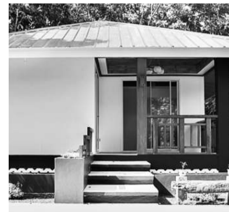
One of the pilot homes built by Strawture Eco in Gorakhpur
