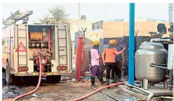
Fire department personnel at the Nuh plant. ■ SPECIAL ARRANGEMENT
