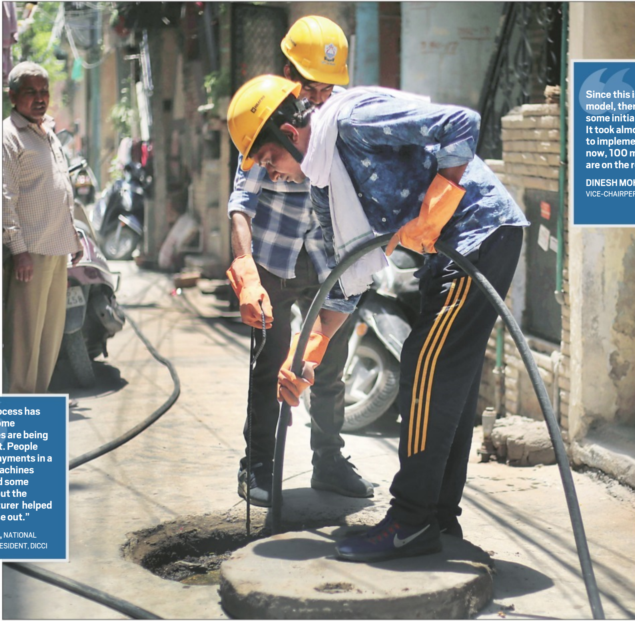
At Mukherjee Nagar's Nehru Vihar, a three-member team attends to a sewer blockage complaint. The sewer cleaning machine is mounted on six-foot-wide blue, green and white mini-truck, which comprises a tank, pipes and an external power source on the bed. Photos: Tashi Tobgyal
