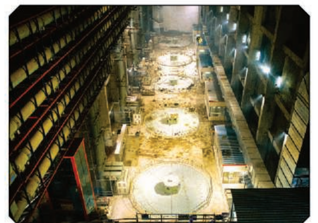
THE PACKAGE - 8 PUMP HOUSE
