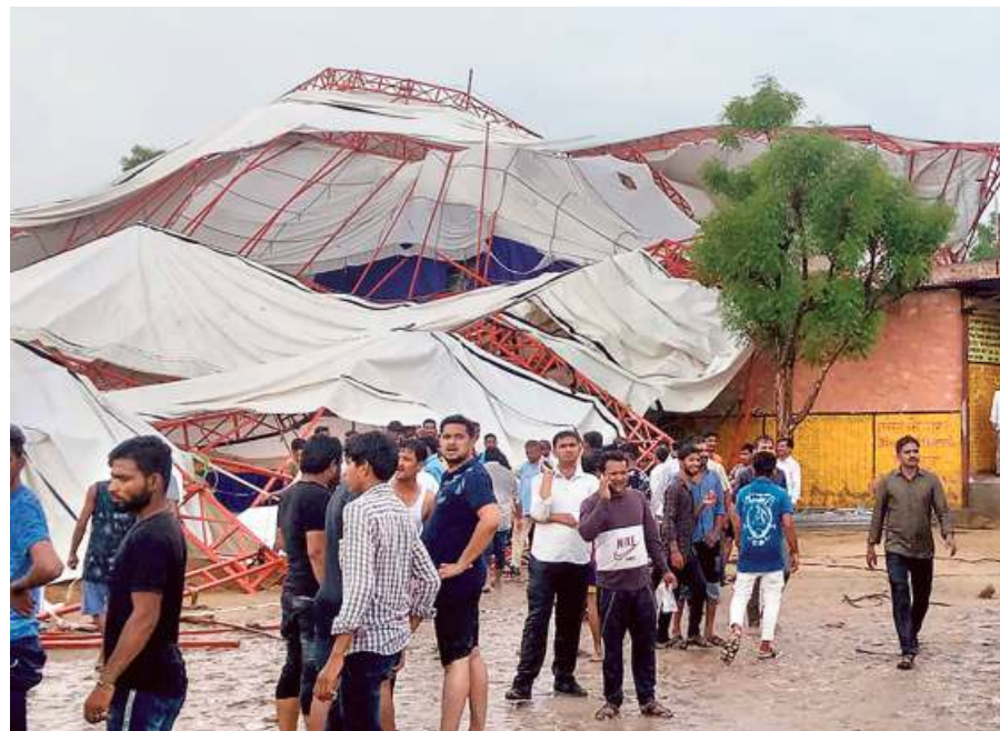
Caught unawares: A pandal, where people had gathered for a 'Ram Katha', collapsed at Jasol in Rajasthan's Barmer district on Sunday after sudden rain and squall. •PTI
