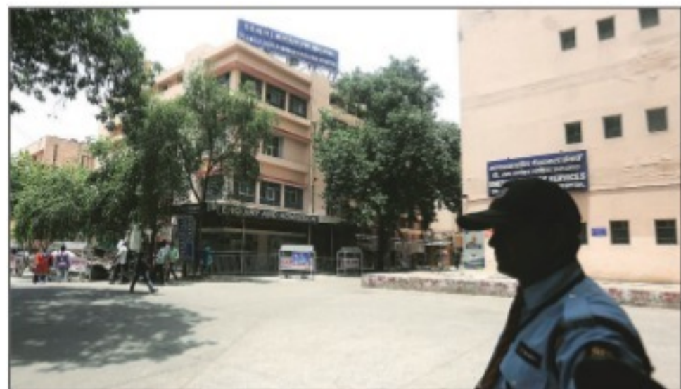
The NDMC will construct the 300-bed super-specialty wing of Ram Manohar Lohia Hospital at Moti Bagh
