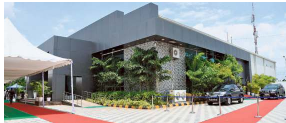
Awaiting demolition: The Praja Vedika at Undavalli near Vijayawada. ■ CH. VIJAYA BHASKAR
