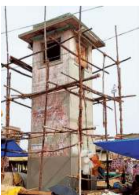
The JFK Memorial Tower Clock under renovation in Chittoor district.
