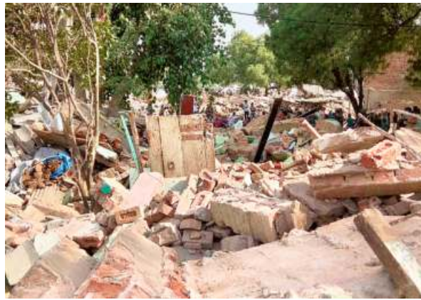
Government officials on Thursday demolished 26 houses in Bawana. ■SPECIAL ARRANGEMENT
