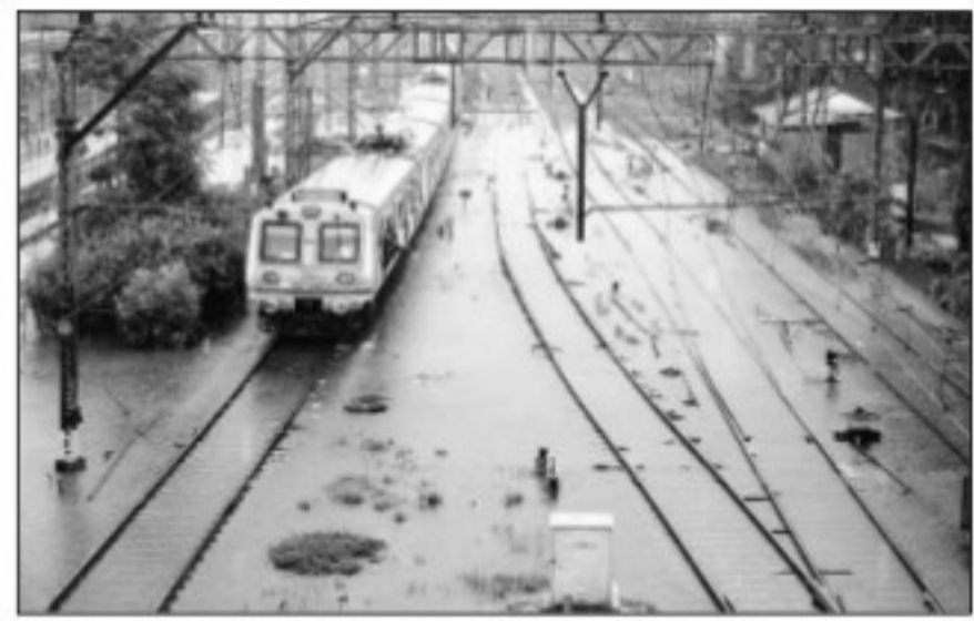
Three people were killed in separate incidents as the first spell of heavy rain lashed Mumbai on Friday. Five others were injured. Deepak Joshi
