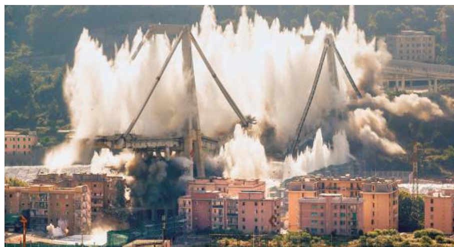
Done and dusted: A cloud of dust rises as the remaining spans of the Morandi bridge, which collapsed nearly a year ago killing 43 people, were demolished in Genoa, Italy, on Friday. AP
