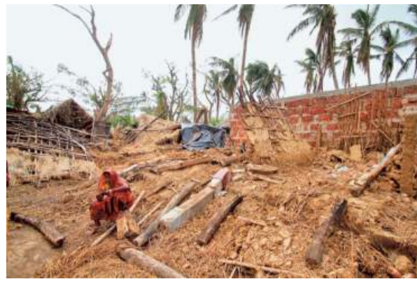
All that remains: A woman from a Dalit family sits near her damaged mud house. • BISWARANJAN ROUT
