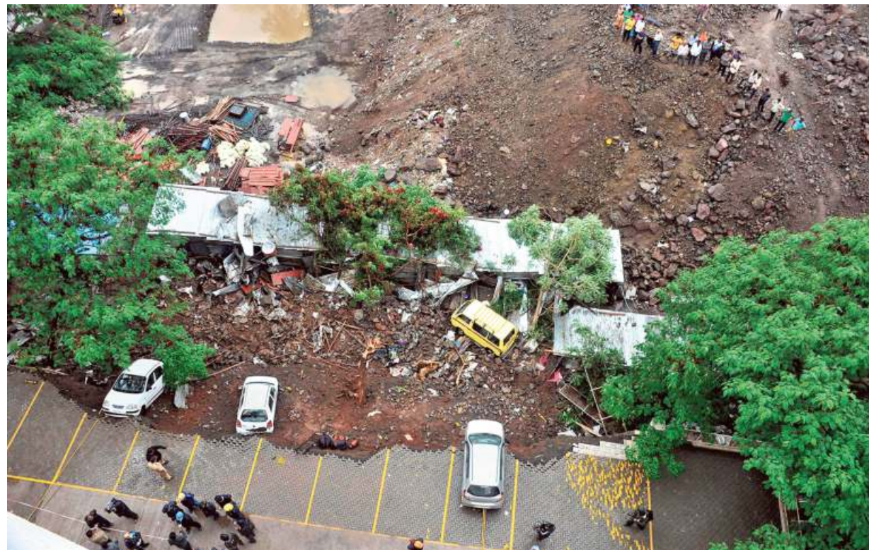
Buried under: As rain pounded Pune, 15 persons, including four children, were killed when a part of a compound wall of an apartment complex crashed on workers' hutments at Kondhwa on Saturday. The deceased hailed from Bihar. *PTI (PAGE 9)
