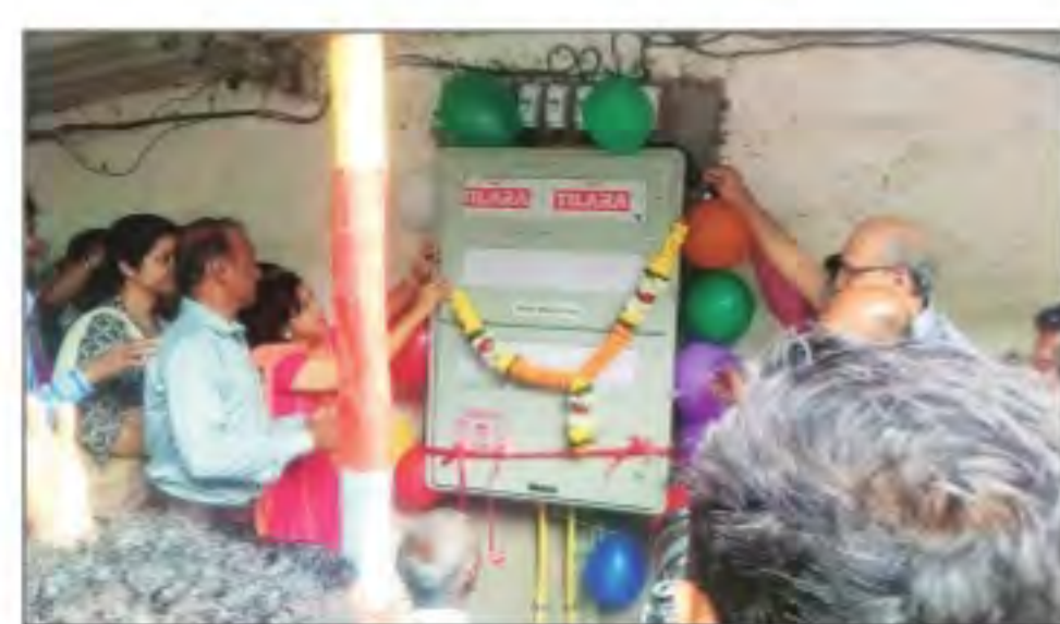
A Mumbai resident chipped in with nearly Rs 2 lakh to help residents clear the funding hurdle to get electricity
