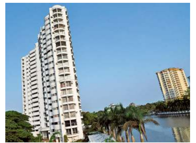
Hopes shattered: Holy Faith apartments and Alfa Ventures (right) are among the five buildings at Maradu in Ernakulam that were ordered to be razed. ■ THULASI KAKKAT
