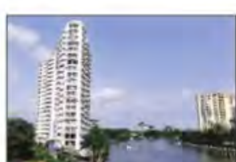
4 apartment complexes are to be razed for CRZ violation
