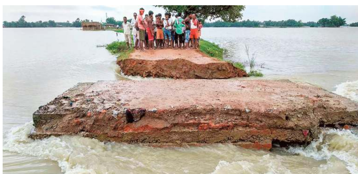
Bihar on alert: People looking at a culvert which was washed away by flood waters at East Champaran in Bihar on Saturday. The Water Resources Department has issued a high alert in vulnerable districts, particularly those bordering Nepal, as water level continues to rise in several rivers in the State following heavy rain in the past six days. PTI
