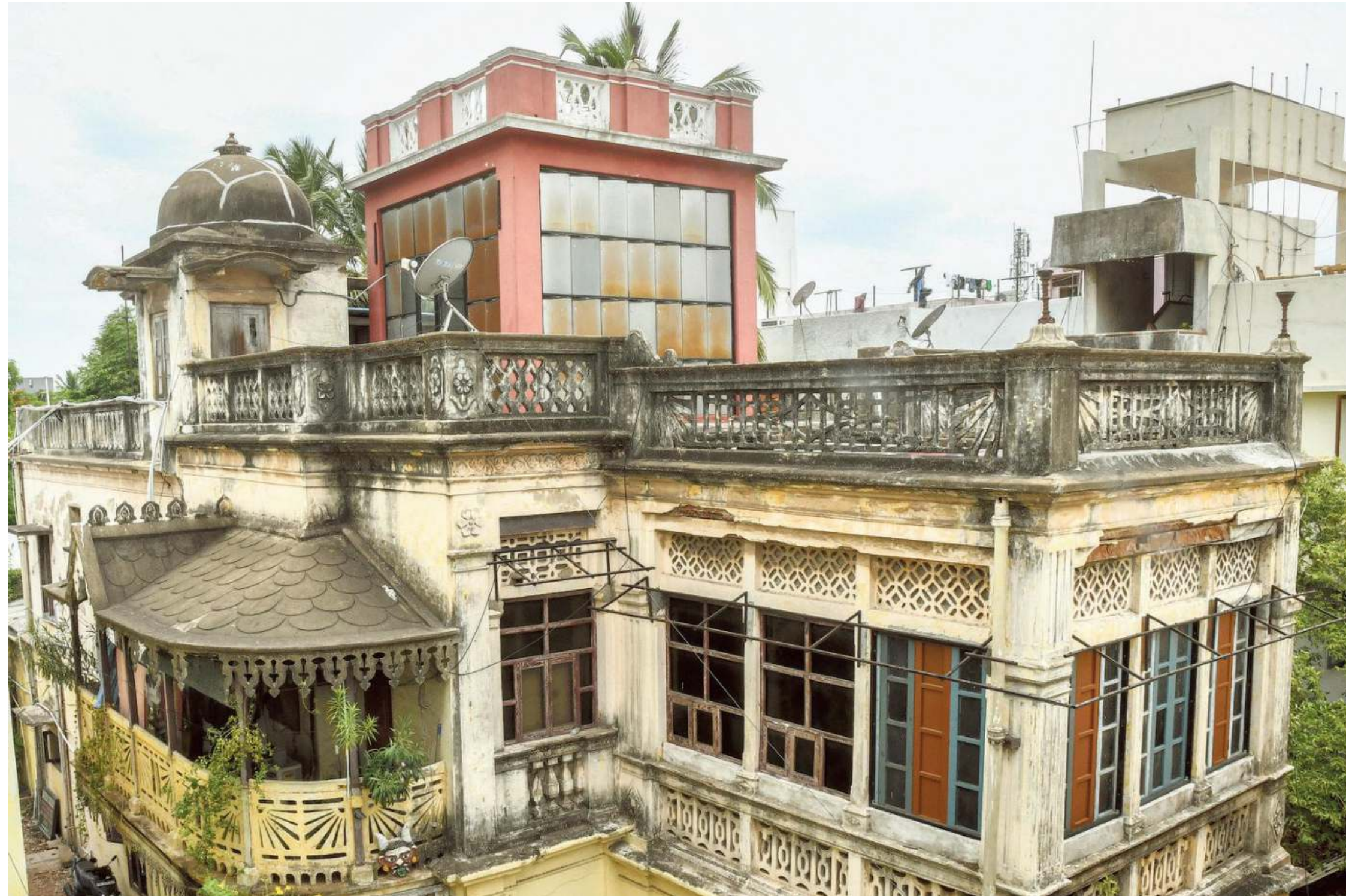
Old is gold Karpaga Vilas in Kodambakkam was once called the airplane house because the portico looked like the nose of an aircraft. Identical ornate balconies on either sides are the wings and the backyard is the tail. R. RAVINDRAN
