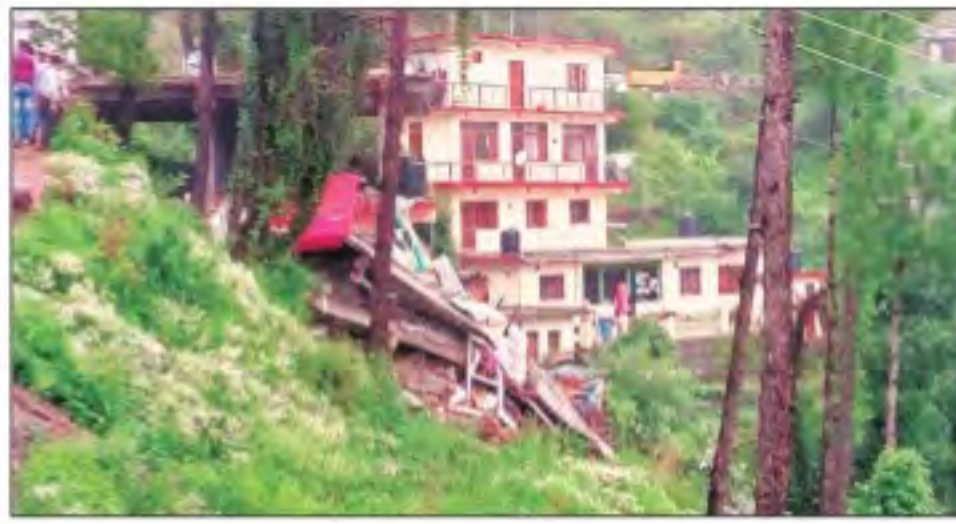
Soldiers of the 4 Assam Regiment had come to an eatery in the three-storey building. Pradeep Kumar
