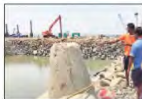
At site of the Rs 12,000-cr coastal road project. File
