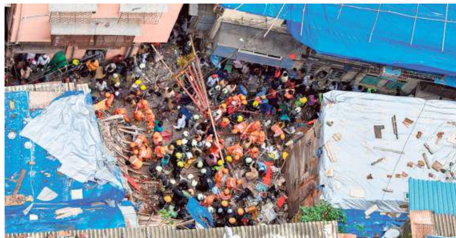
Reduced to rubble: NDRF personnel and rescue workers searching through the debris of the building that collapsed in Dongri, south Mumbai, on Tuesday. • VIVEK BENDRE
