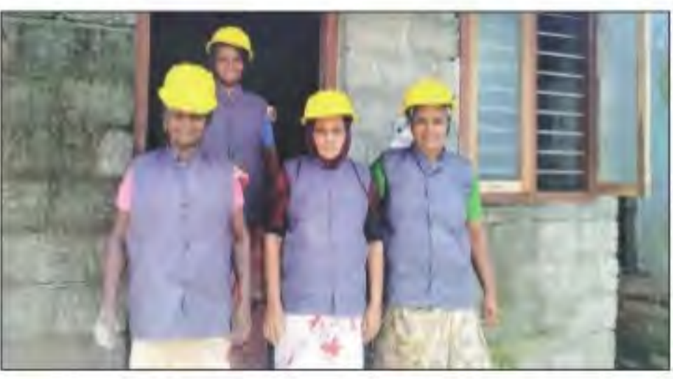
Sicily (left), 74, and the other members of her construction team at site of their latest project in Kumbalangi. Vishnu Varma
