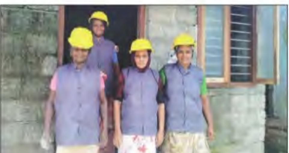
Sicily (left), 74, and the other members of her construction team at site of their latest project in Kumbalangi. Vishnu Varma
