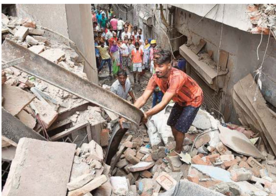
An abandoned four-storey building collapsed in central Delhi's Nabi Karim on Wednesday. No one was injured in the incident. ■SUSHIL KUMAR VERMA
