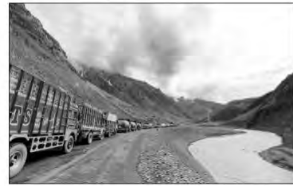
A traffic jam near Manimarg on the Srinagar-Leh highway on Saturday, after landslides hit Zojila pass. Shuaib Masoodi
