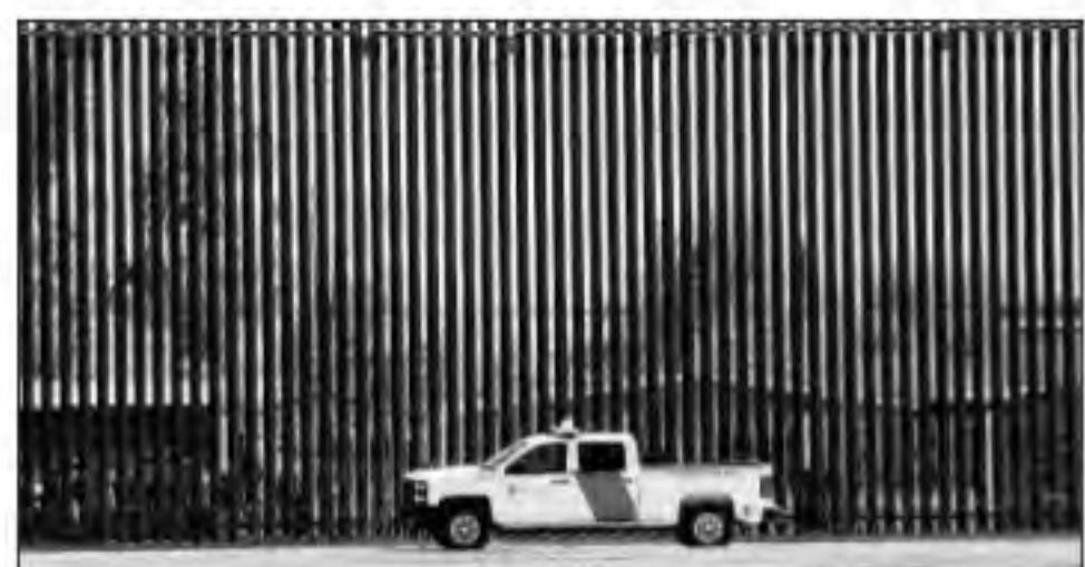
A portion of the border wall in El Centro, California. File
