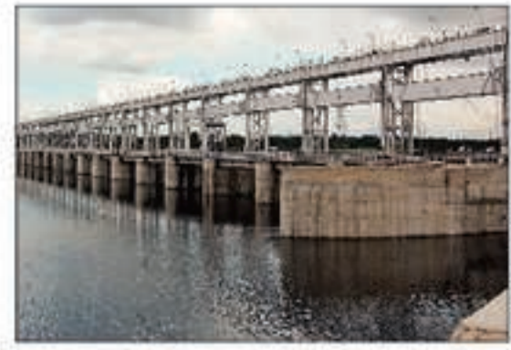
379 MW. These are GMR's Bajoli Holi project in Himachal Pradesh with a total capacity of 3x60 MW, L&T's Singoli Bhatwari project in Uttarakhand with a total capacity of 2x33 MW and Soranghydel project with a proposed capacity of 2x50 MW at Uttarakhand.
