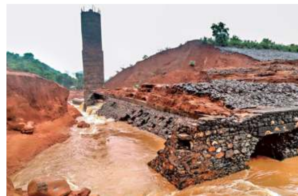
Force of nature: Water flowing out of the breached Tiwara dam in Ratnagiri district of Maharashtra. • RAJU SHINDE
