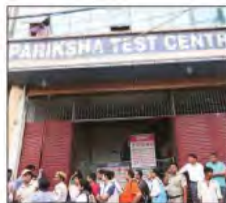
The centre where the fire broke out. Gajendra Yadav
