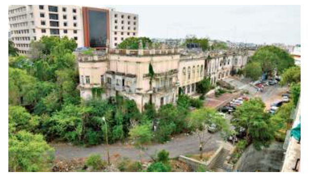
Errum Manzil Palace in Hyderabad that is proposed to be razed to make way for the Assembly building. ■ FILE PHOTO
