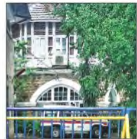
ATS office in Mumbai
