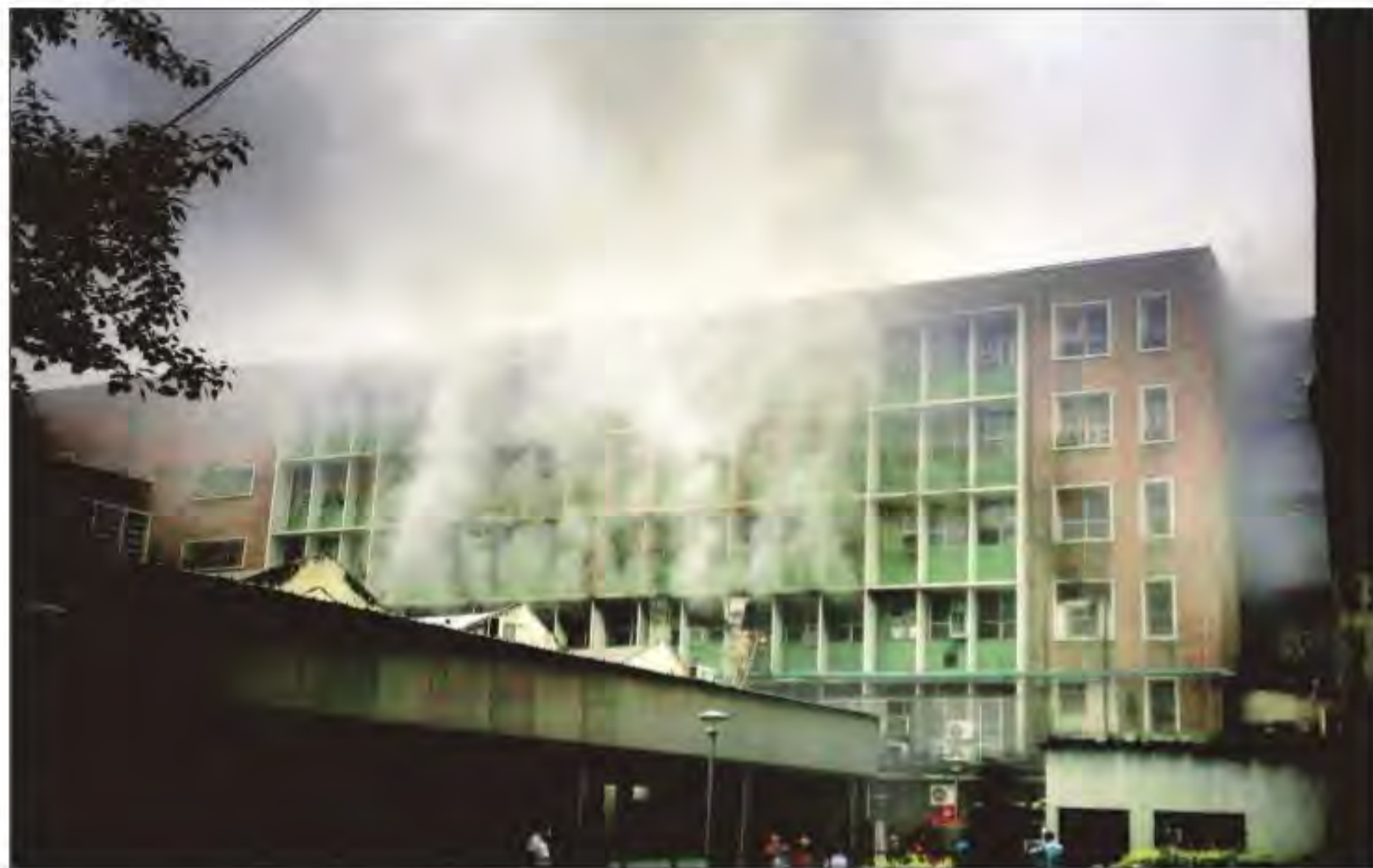
The fire started on the second floor of the teaching block at AIIMS and gradually spread to the third, fourth and fifth floors of the building. Praveen Khanna
