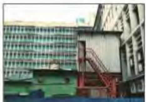
Fire officials said the temporary structure houses diesel generator sets
