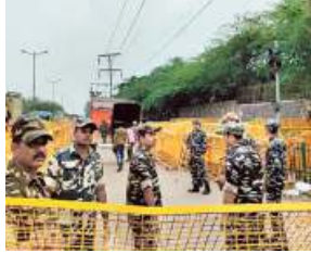
CRPF officers at the site where the demolition was carried out in Tughlakabad Extension, on Thursday.
