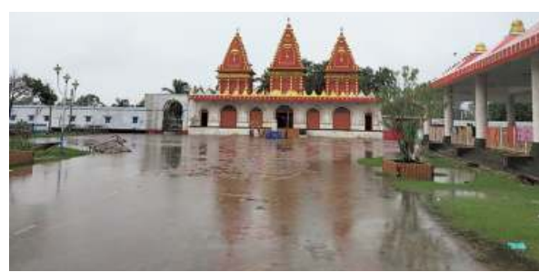
Closing in: The temple is facing the threat of submersion in the next few years. ■ SPECIAL ARRANGEMENT
