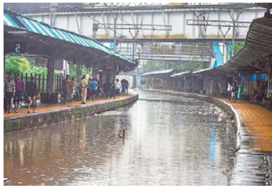
Closed line: The tracks at the Chunabhatti station in Mumbai went under water on Sunday. ■PTI
