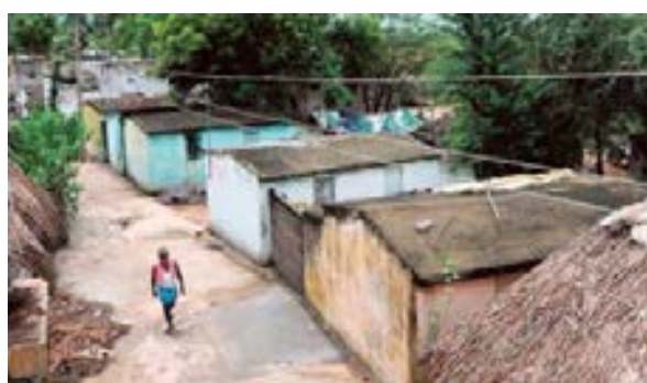
The rural housing scheme aims to ensure every rural Indian family has a pucca house with basic amenities by 2022.
