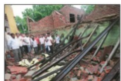
2 kids died when a house collapsed in Rabupura, Monday night. Gajendra Yadav
