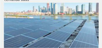
71.41 KW Projected annual system output: 86,244 kWh (equals to carbon dioxide 30,246 Kg of coal burned or carbon sequestered from 1,008 tree seedlings
