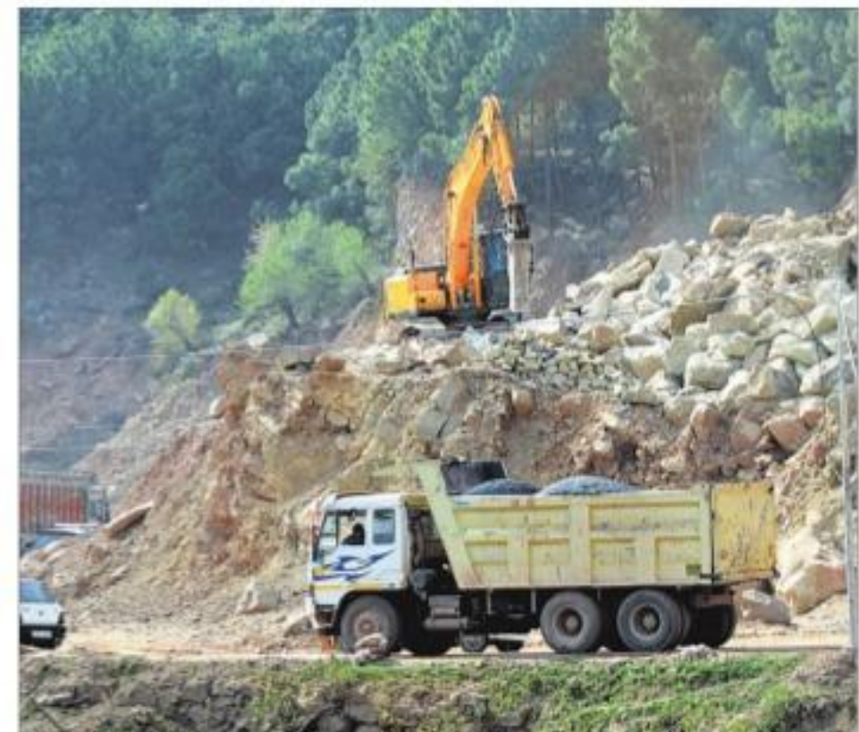
Four-laning under way on the Jammu-Srinagar highway. FILE
