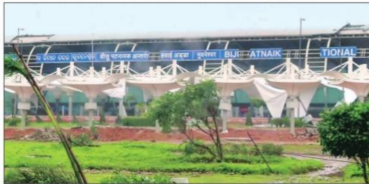
The Biju Patnaik International Airport in Bhubaneswar during Cyclone Fani earlier this year. The World Bank estimates the damage caused by Fani at $4 billion. ANI
