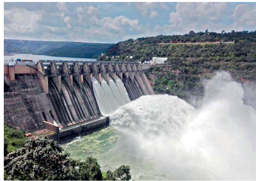
Four crest gates of Srisaillam dam was opened on Sunday after water in the reservoir recorded 884.80 feet against the total reservoir height of 885 feet.
