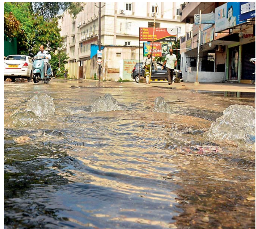
Overflowing water gushes from clogged drains at Vidyanagar even as the area is inundated with rainwater.
