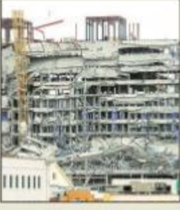
The partially collapsed Hard Rock Hotel in New Orleans. AP
