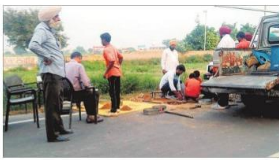
Officials inspect a road in Fatehgarh Sahib. TRIBUNE PHOTO
