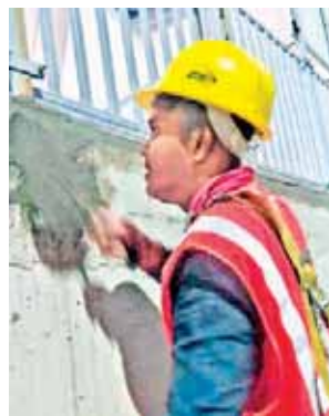
works every day from midnight to early morning without obstruction to traffic. "All parts of the station areas
