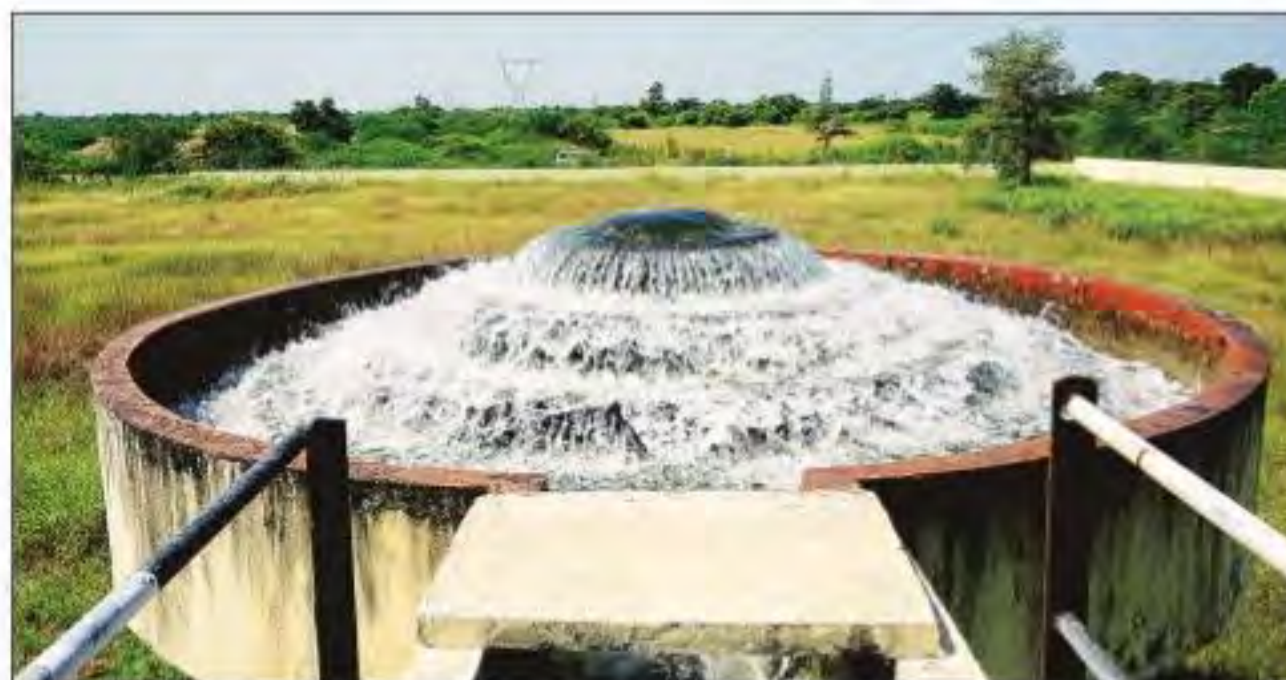
A water filtration plant of Waghodia taluka of Vadodara district Bhupendra Rana
