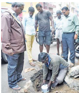
Officials close unused borewell on Saidapet main road in Vellore on Tuesday. Totally 15 borewells closed. — DC
